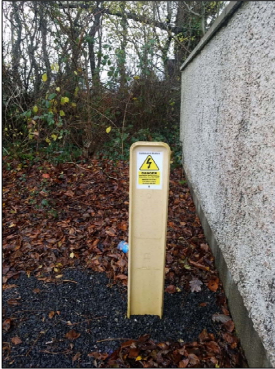
Plate 10-5 View of existing cable road post that runs under the small road that connects the south substation to the cable route.
