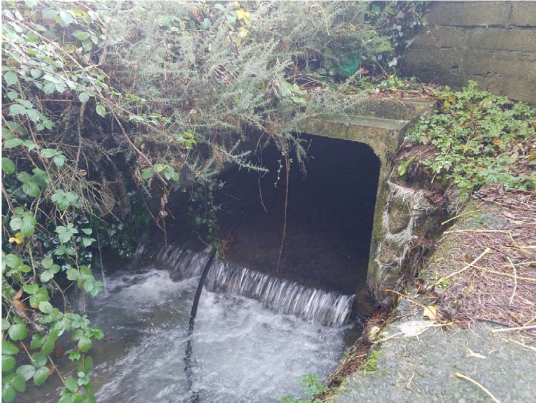
Plate 3.10 View of box culvert on Borris Stream. Directional bore was used to install cable under culvert.
