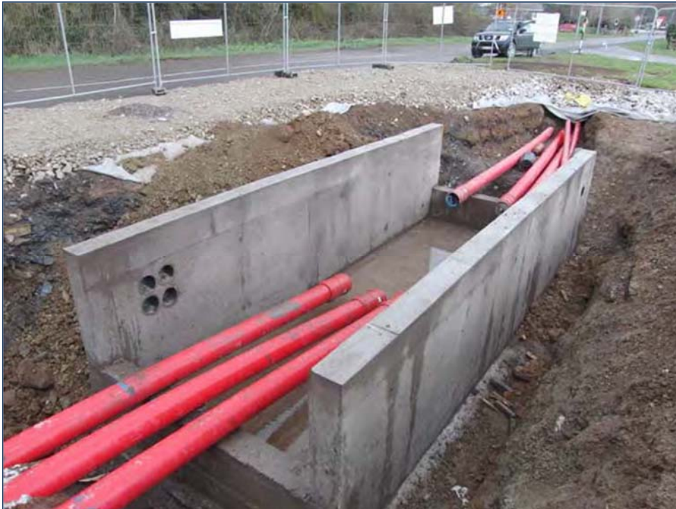
Plate 3.5 Typical joint bay construction, adjacent to public road (generic example).
