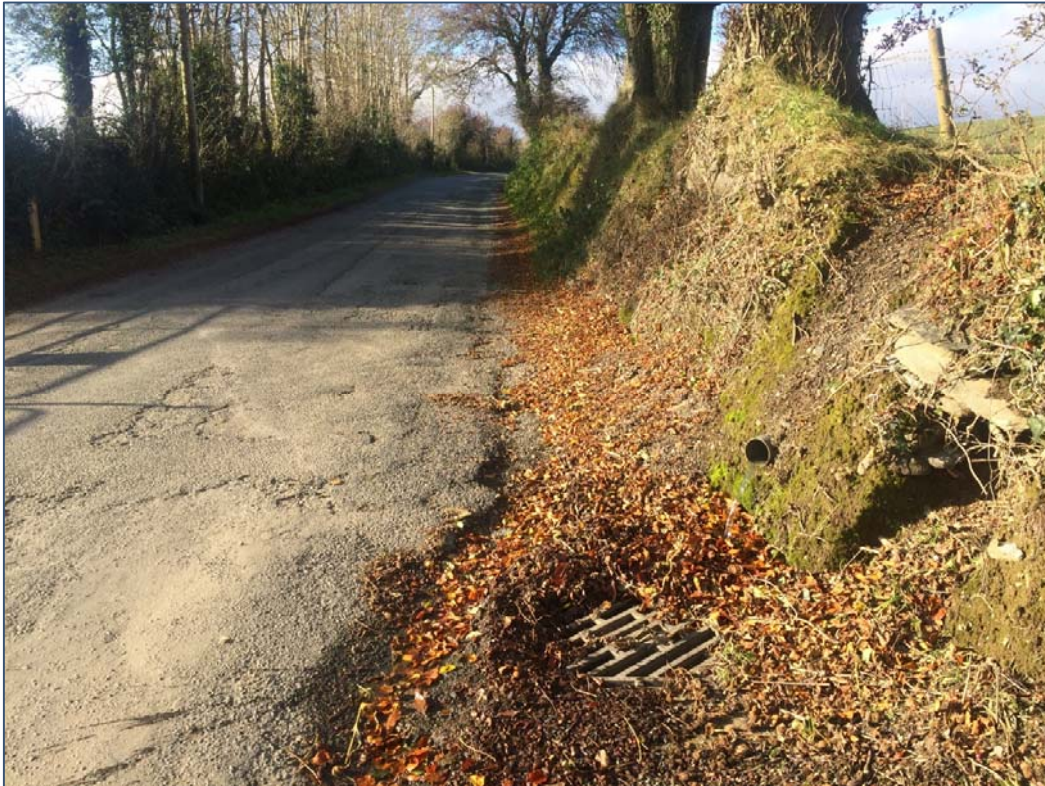
Plate 3.6 View of current, post construction conditions at typical storm drainage pipe crossing location
